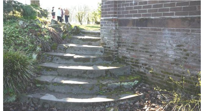
Poorly repaired steps beside a former rockery and raised wall, Halecroft Park
