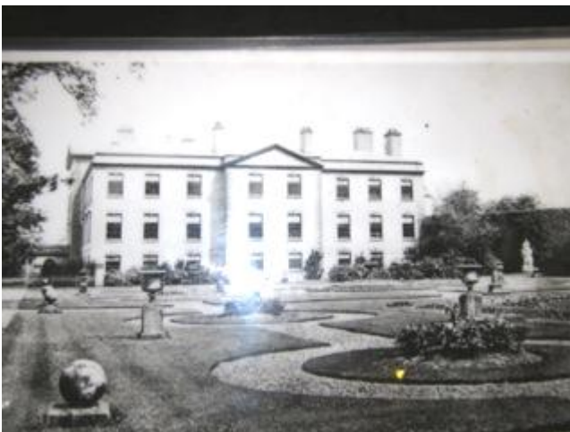
South elevation with formal garden c. 1900
